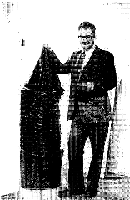
Here Eb Rice poses with piles that have "come to grief" in encounters with ice-cemented gravel.
