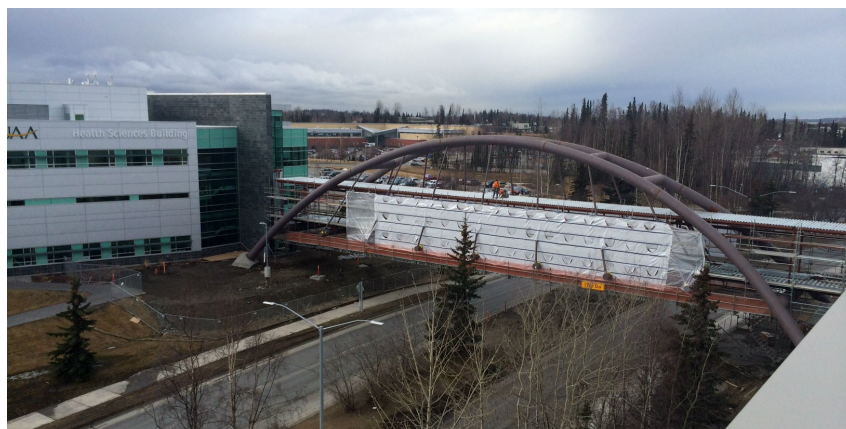
Pedestrian Bridge Construction Has Resumed
